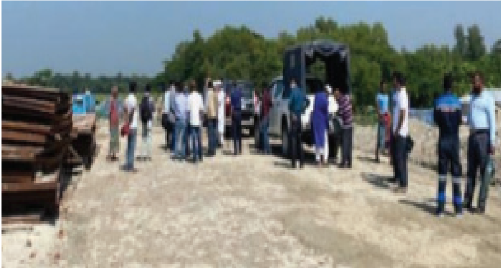
Site visit at construction for the new 15 MW power plant at Hatiya Island
